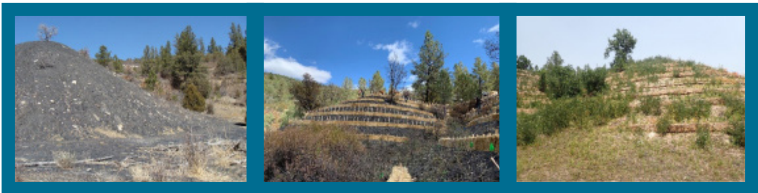
Figure 8 — A coal waste pile before, during, and after the Tin Pan Mine Reclamation Project
